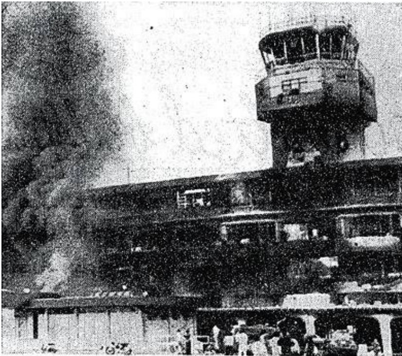
Fig. 5. Terminal of the Manila International Airport was heavily damaged because of a fire from an undetermined origin (1972). The New York Times Archives.
