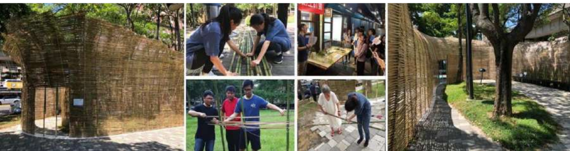
Fig. 9. The actual implementation of bamboo structures as part of course outcomes under the USR program for place-making
