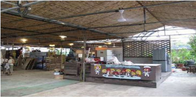
Fig. 6. Open concept greenhouse structures – kitchen area beside SURF site.
